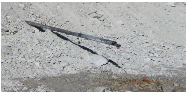
Figure 7. Completed horizontal drainhole with water flow
