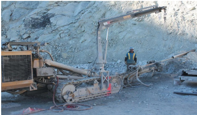
Figure 6. BAT Construction drainhole drill at HVC.
